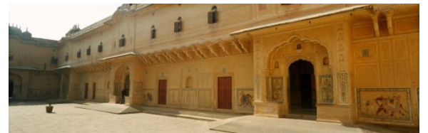
Fig 5.3: Sand stone is widely used in the exteriors
