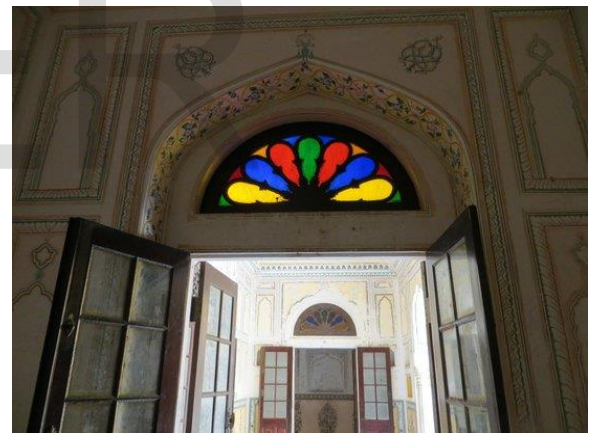
Fig 5.4: Wooden doors & windows with Belgium glass
